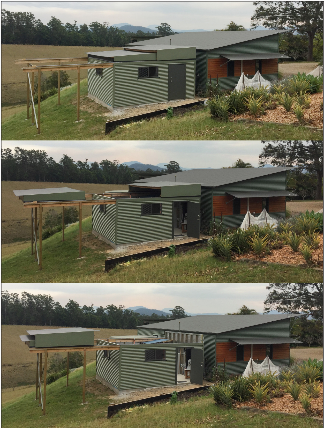
Figure 1. Observatory with roof closed (top), partially open (middle) and fully opened (bottom). To the right of the observatory is a Granny flat (sans Grannies) and double garage.
