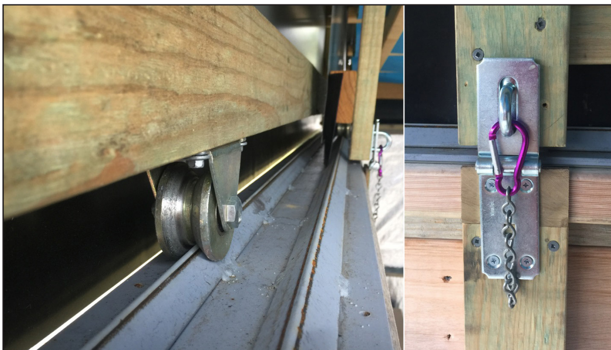
Figure 2 Left. Roof tracks and casters. Right. One of six hasp and staples for securing the roof when closed.
