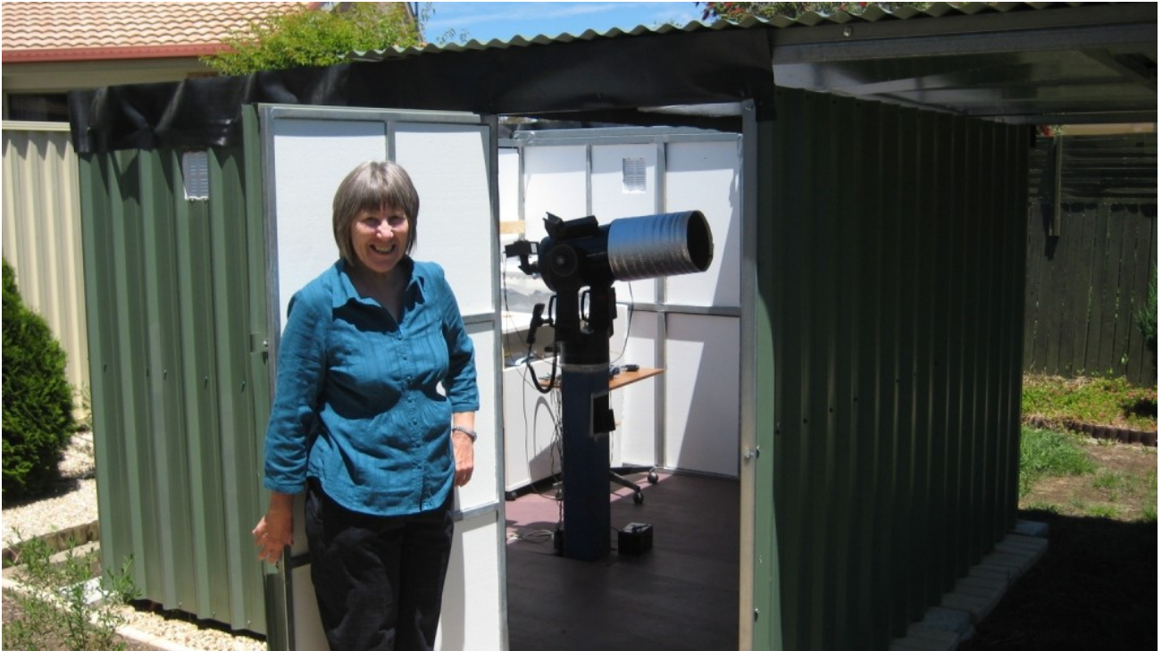
'Lexy's Palace' in Canberra. The walls are galvanised sheeting with styrofoam insulation (one day I'll paint it a darker colour). The roof easily rolls back. The timber floor is suspended on concrete pavers and is discrete from the pier cemented into the ground.
