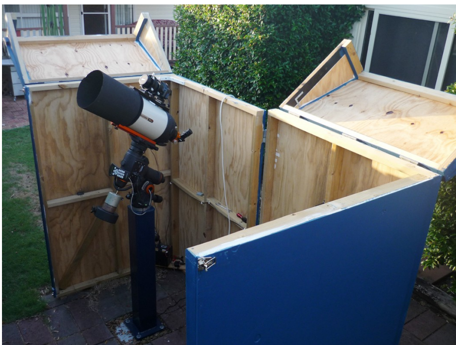
Figure 1. The observatory from which Mark observes. The Canon 450d camera can be seen mounted piggyback on top of the telescope. Space restrictions required a novel solution to the problem of permanently mounting the telescope. The long wall is hinged in the middle and the end wall nearest the camera is equipped with wheels allowing it to easily swing round to enclose the pier. The split roof can then be closed to protect the telescope when not in use. When open for observing there is ample room in which to work, inspiring Mark to paint the outside TARDIS blue. However, when closed, friends have compared it, rather unkindly, to an outhouse.
