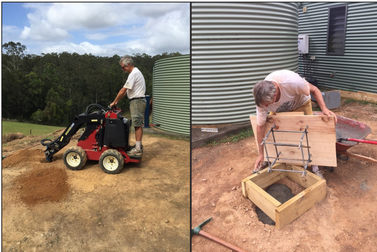
Figure 2. Left: a post-hole digger made light work of the two pier holes. Right: frames made from welded lengths of galvanized threaded rod were cemented into each of the pier bases.
