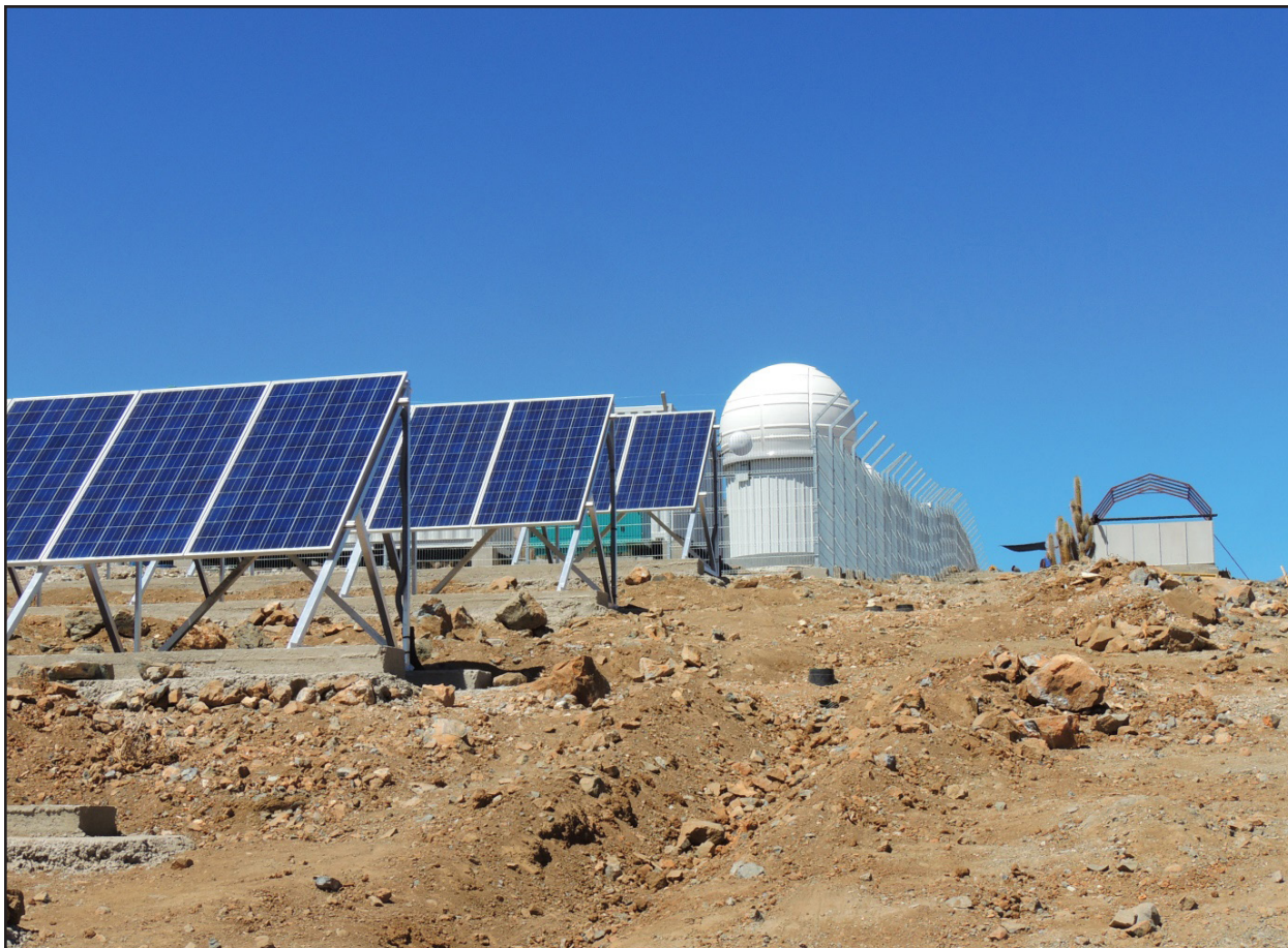
The solar panel installation at El Sauce. The dome is in the Russian sector of the site.
