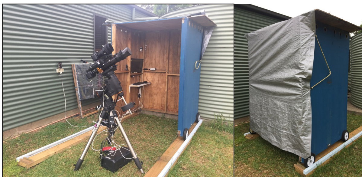
Figure 1. Left: Original Sydney observatory was transformed into a roll-off shed design as a temporary shelter whilst the permanent roll-off roof observatory is constructed. Right: A tarpaulin fixed in place with Occy straps provides adequate weatherproofing.
