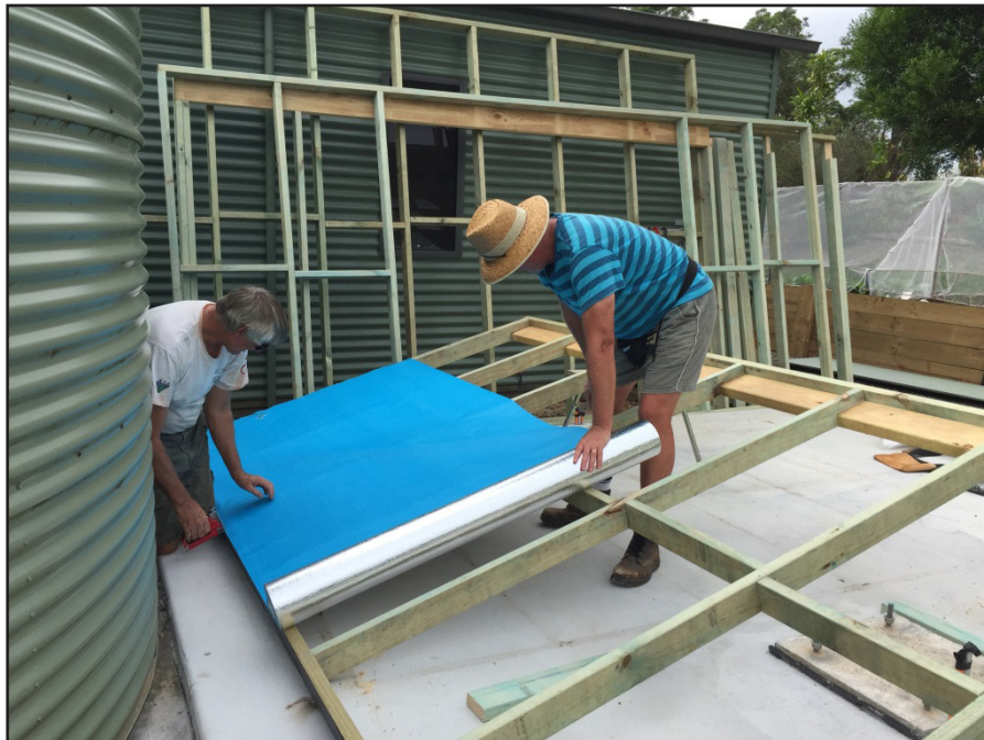
Figure 1. Danny and I installing insulation foil to the west wall before attaching corrugated iron sheeting and lifting the wall into place.
