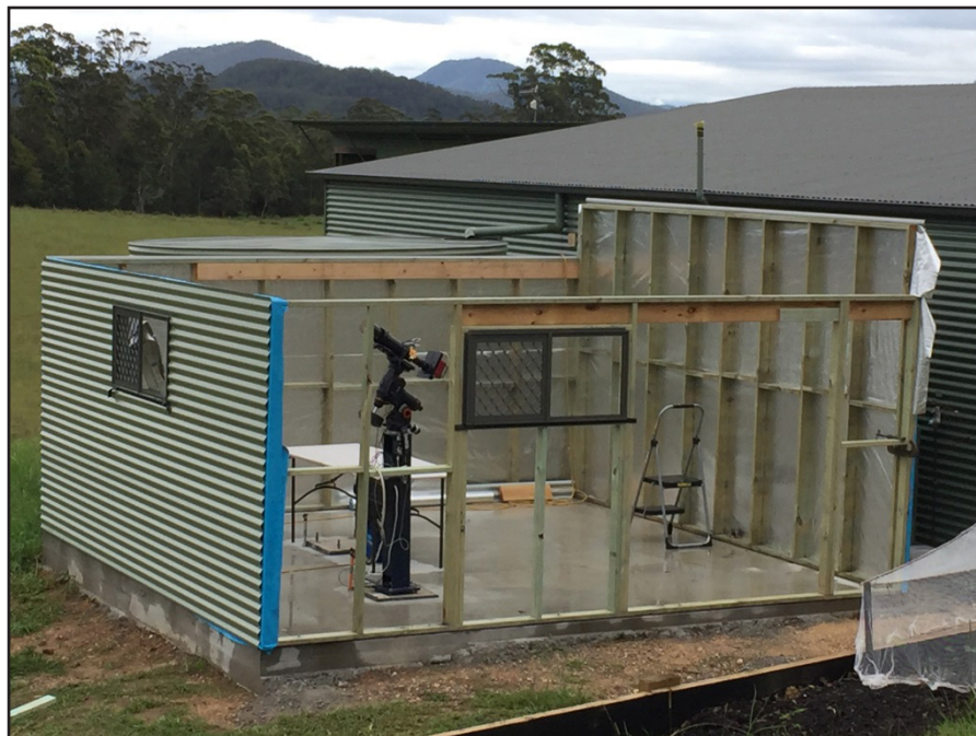
Figure 2. Building mostly erected, with one telescope installed.
