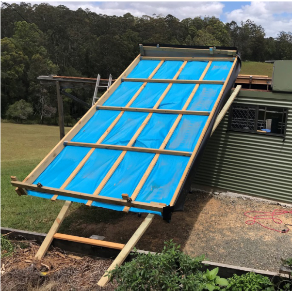
Figure 3a. Removal of roof section
