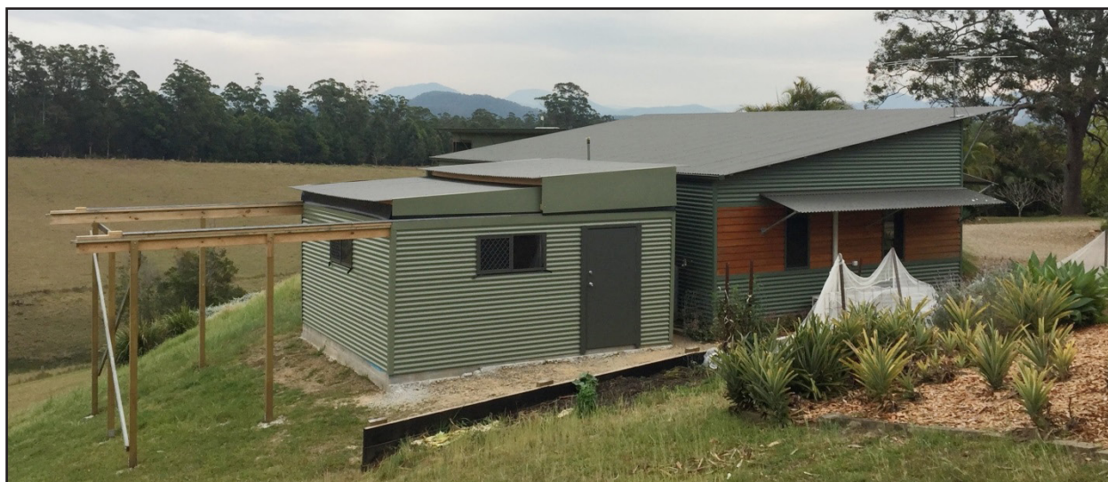
Figure 1. How the roof sections should look.
