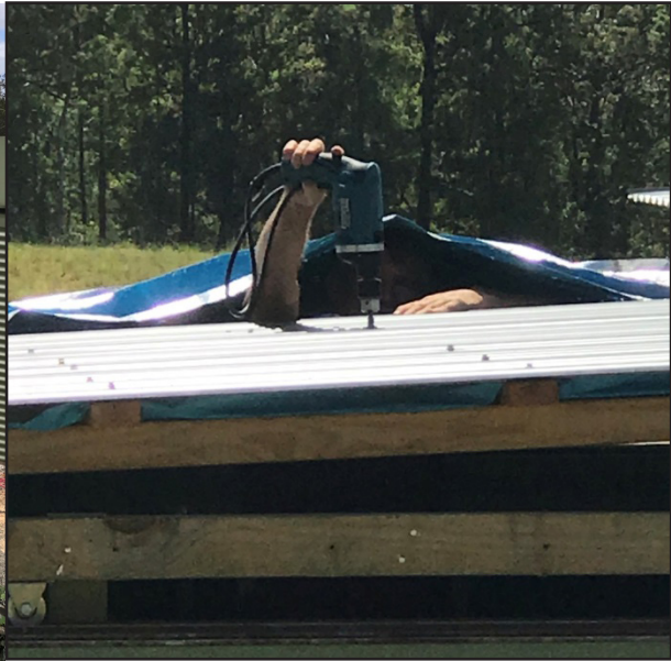
3b reinstallation of colorbond sheeting
