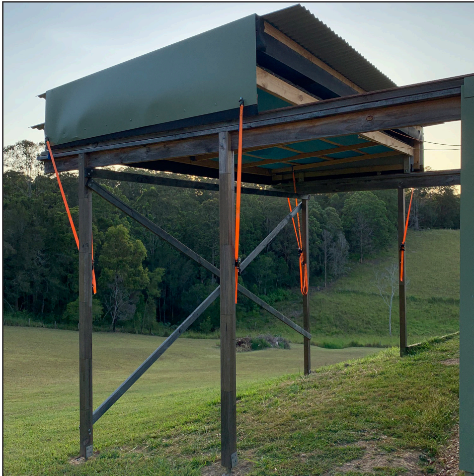
Figure 4. Roof sections secured in closed and open positions.
