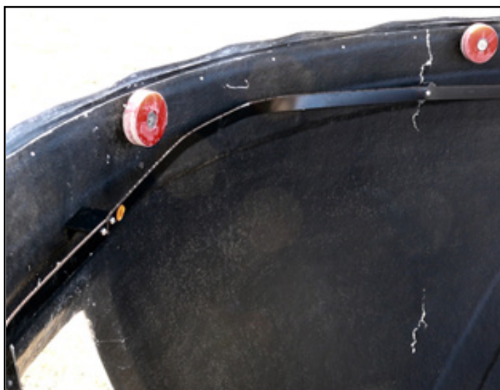
Left. The steel track for dome rotation was twisted in several places. Right. The dome slit cover track was partly torn off at the base.
