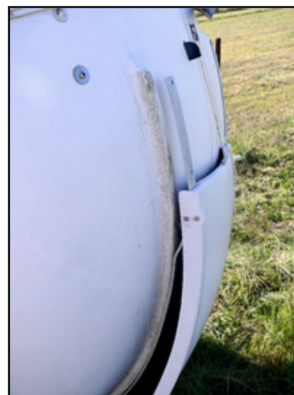
Left. The steel track for dome rotation was twisted in several places. Right. The dome slit cover track was partly torn off at the base.
